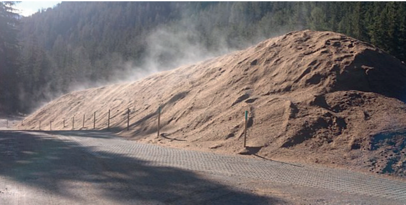
Snow storage in Davos under a protective layer of sawdust.
