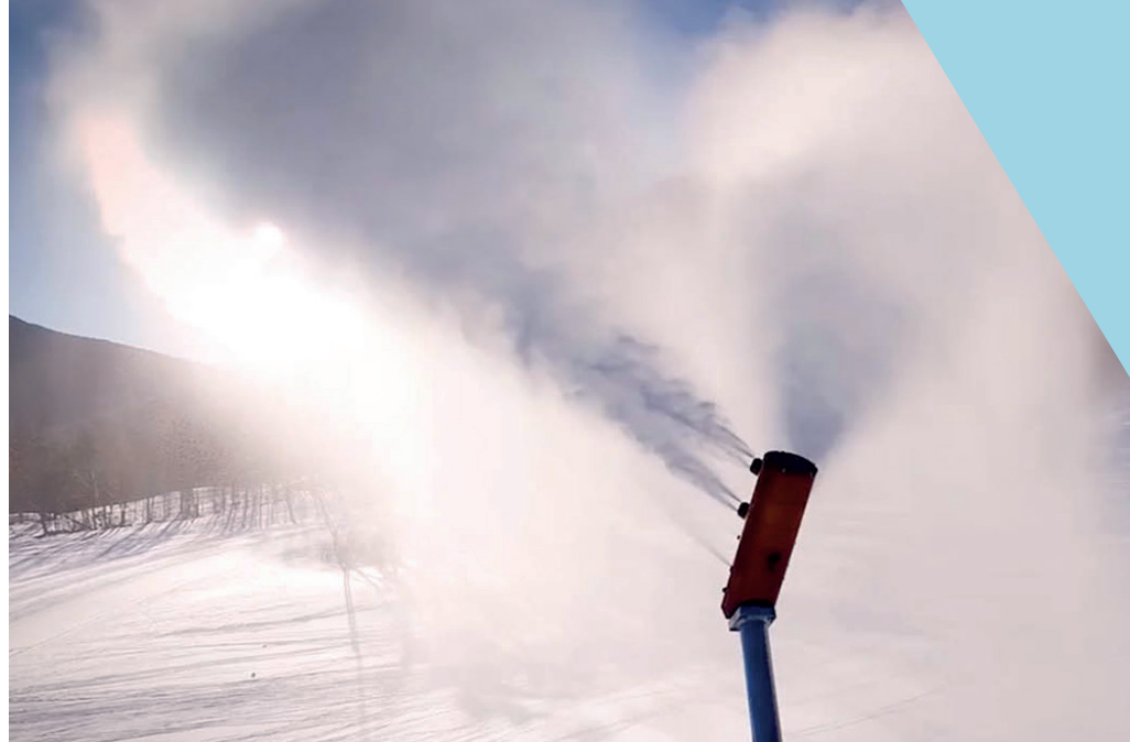
An example of an automatic snow pole connected to a fixed water distribution network.
